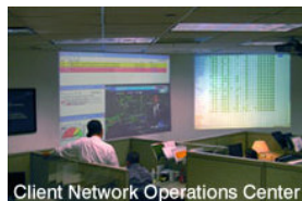
Client Network Operations Center
